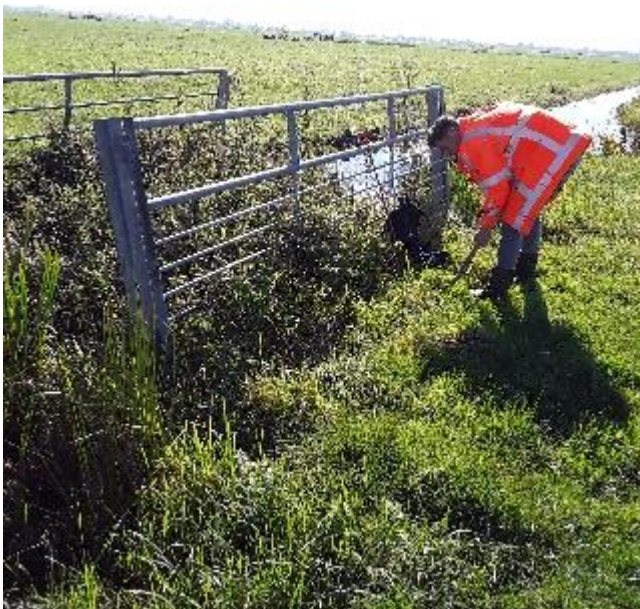
Foto's dam VD18
