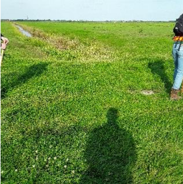
Foto's dam VD11
