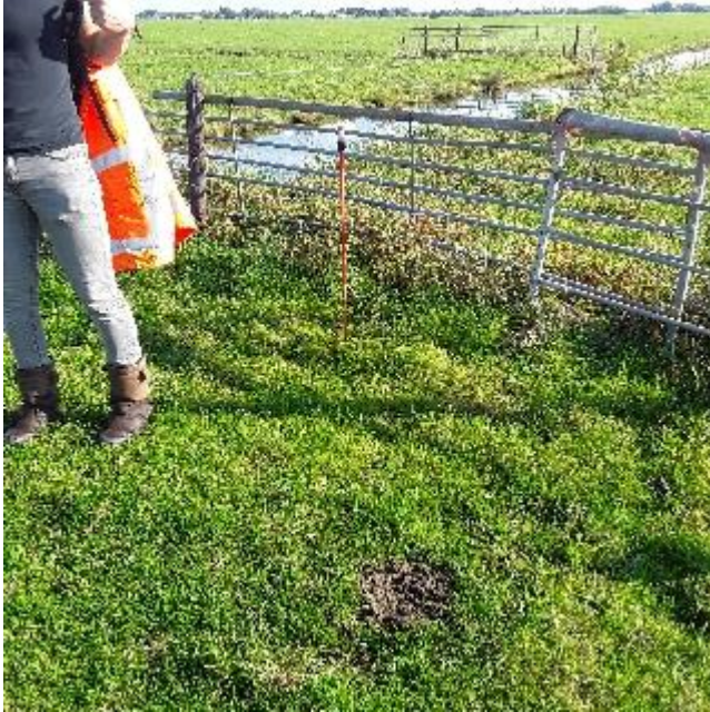
Foto's dam DB14
