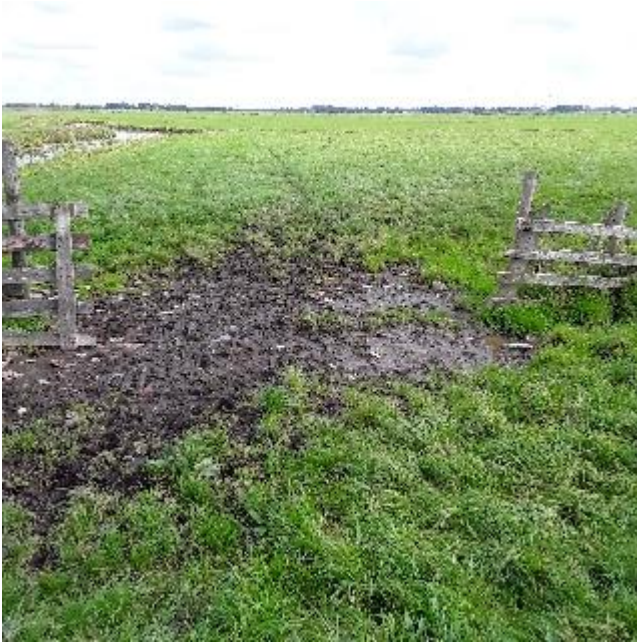
Foto's dam VD28
