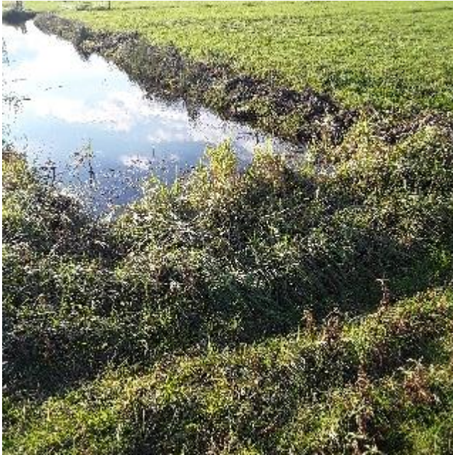
Foto's dam DB17
