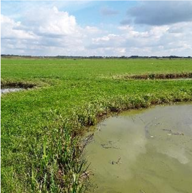
Foto's dam DB10
