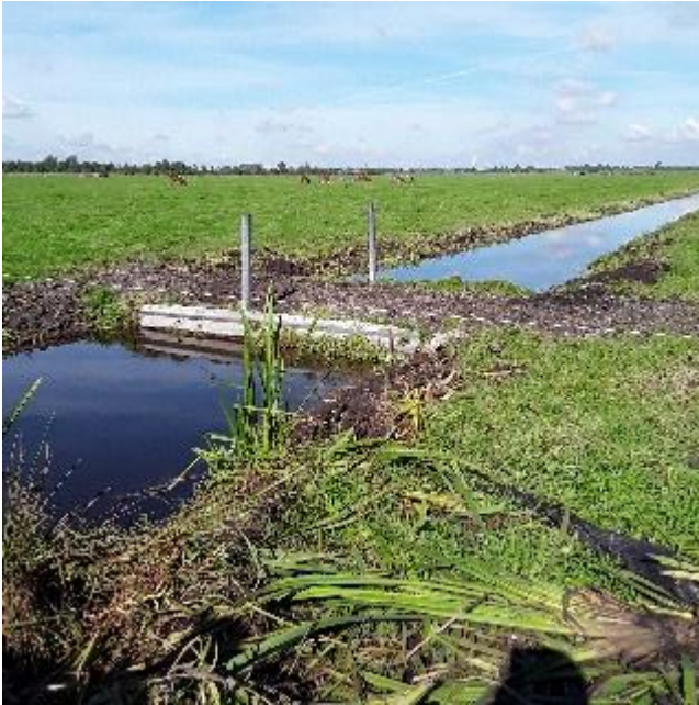
Foto's dam DB08
