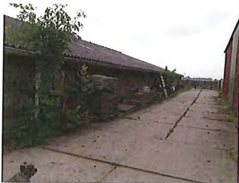
Foto 1: te slopen stal (600 m2)
