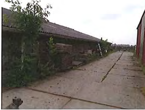
Foto 1: te slopen stal (600 m2)
